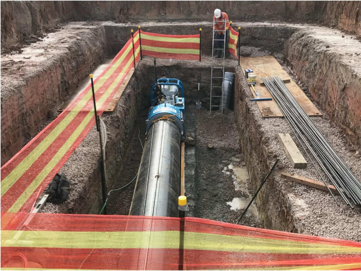
FIGURE 1.2 – REFERENCE IMAGES OF 'BORTEC' BORING MACHINE
