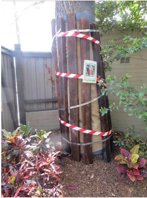
Figure 9. Example of trunk protection
