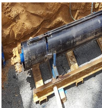
Cutter head and horizontal steering head ground
