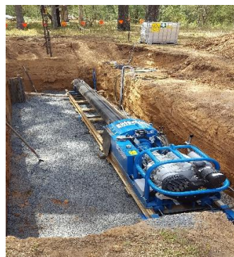
Machine set up on rails
