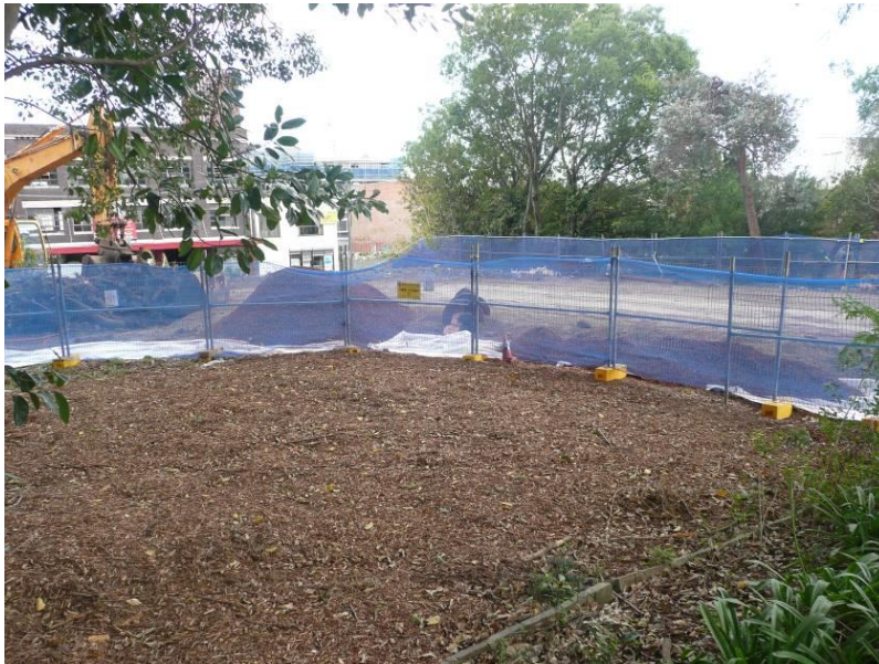
Figure 10. Example of Tree Protection Fencing & mulching requirements
